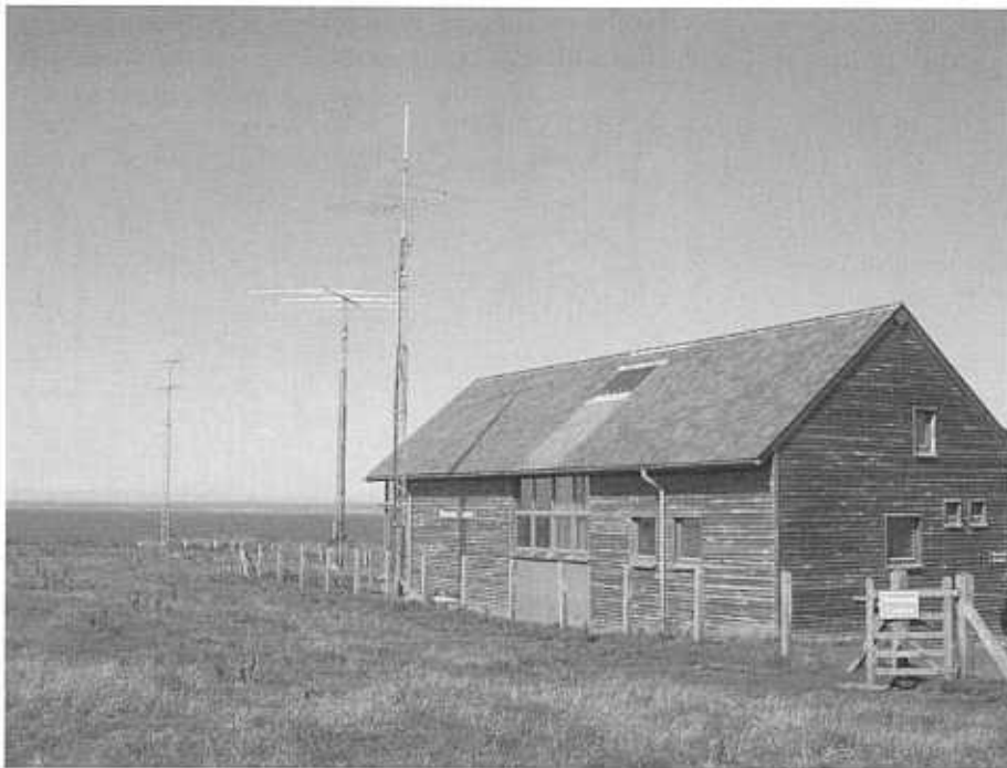
Fig. 2. The Poldhu Amateur Radio Club purpose-built “radio shack” and museum on the National Trust Marconi Historical Site, from which the Beacon GB3SSS and amateur radio station GB2GM operate. (Photo Bart Lee).
