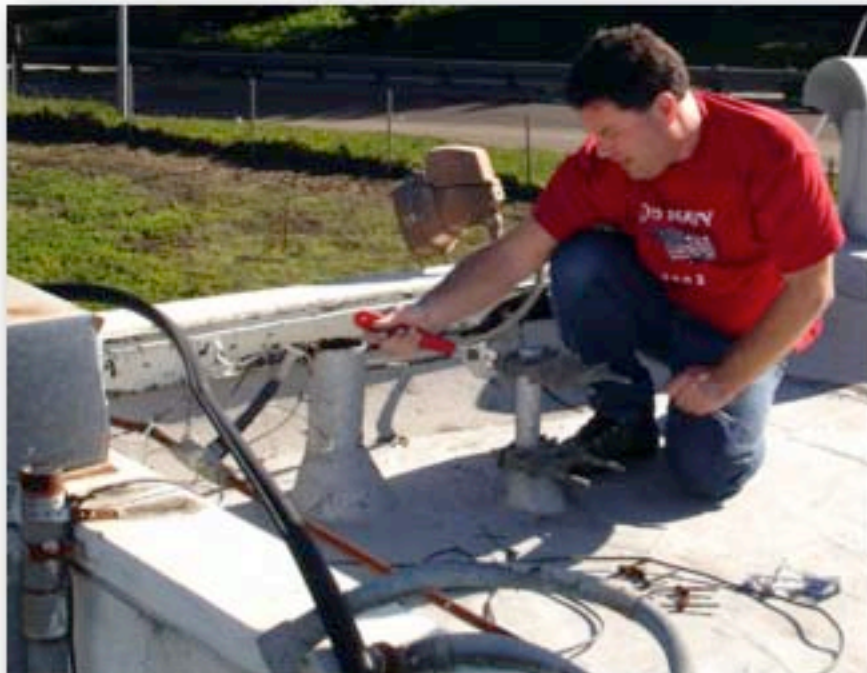
Paul Shinn installs the W6CF/B beacon antenna
