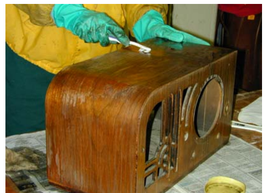
Figure 9: Using an old toothbrush for trim, corners, and detail areas.
